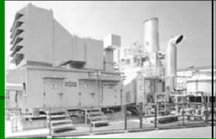
Co-generation system (Kyoto Plant)
