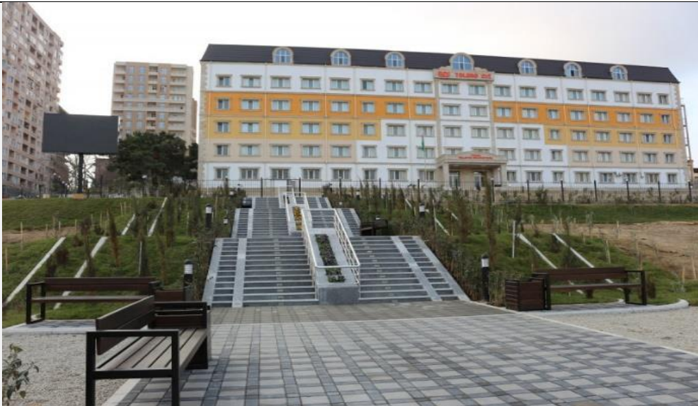
New five-story student's dormitory
